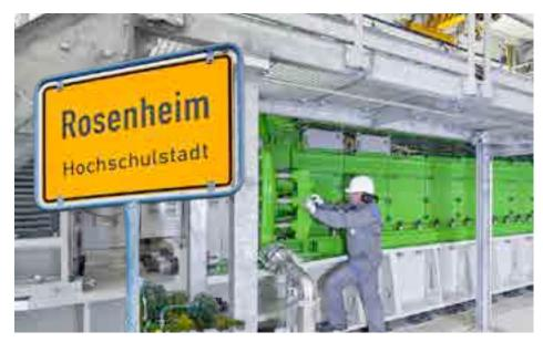
The J920 FleXtra gas engine adds another 9.5 MWel to the Stadtwerke Rosenheim's installed capacity. Three J620 gas engines (3 x 3.35 MWel) as well as one J624 two-stage turbocharged gas engine (4.4 MWel) were installed in previous years.
