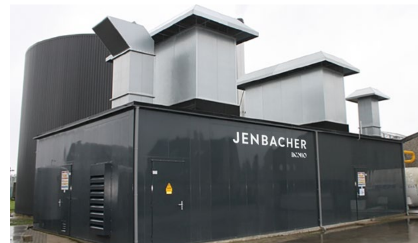
Modular Jenbacher greenhouse CHP solution with acoustical outdoor enclosure
