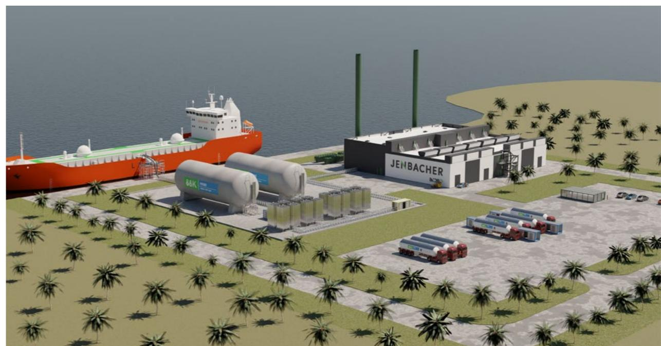
Decentralized power plants typically are in the 10 MW to 50 MW range, which matches our Jenbacher engine product portfolio of 250 kW up to 10.4 MW of single unit electrical power output. Challenges by sea and small island access are easily solved with our engines' compact dimensions and INNIO's containerized solutions, which are quick to install.
